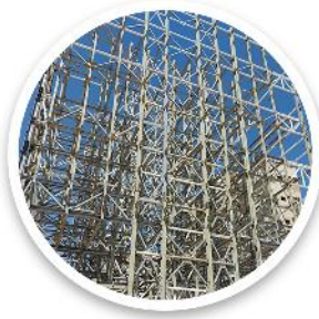
HEAVY DUTY BUILDING
